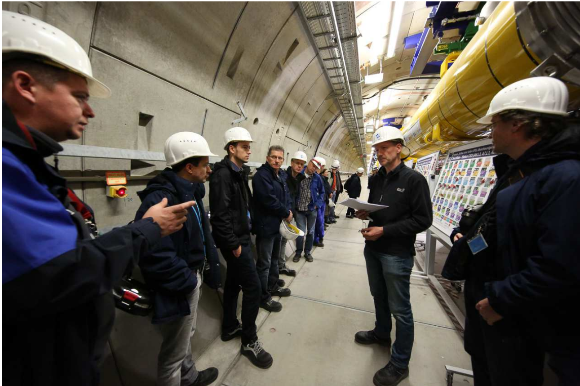
Figure 3. Weekly meeting in the accelerator tunnel at the site of installation.
