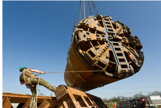
Removing the cutter head \varnothing 5.3m
