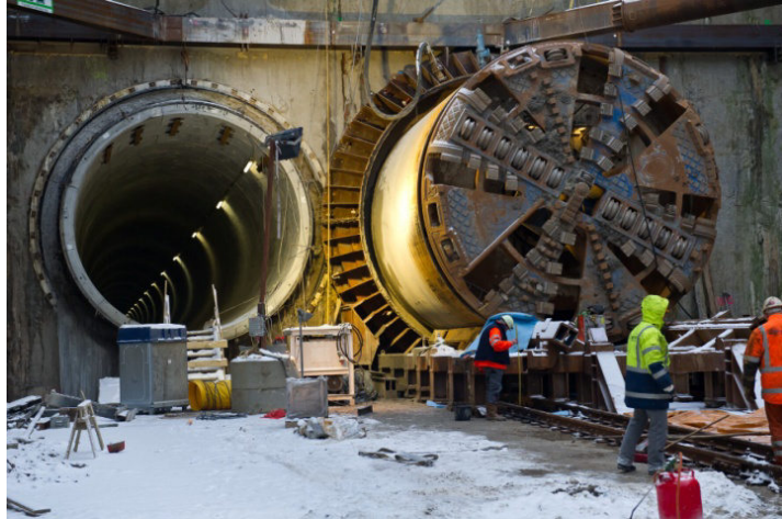
Breakthrough at beam switchyard
