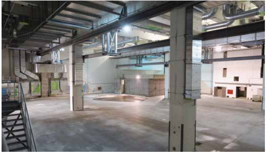
Figure 2 View of XHEXP1 with the final high-precision floor and the HED radiation protection enclosure
