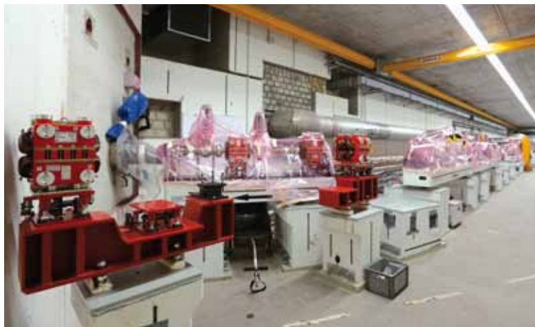
Figure 2 View into the injector tunnel (XTIN) (November 2014)
