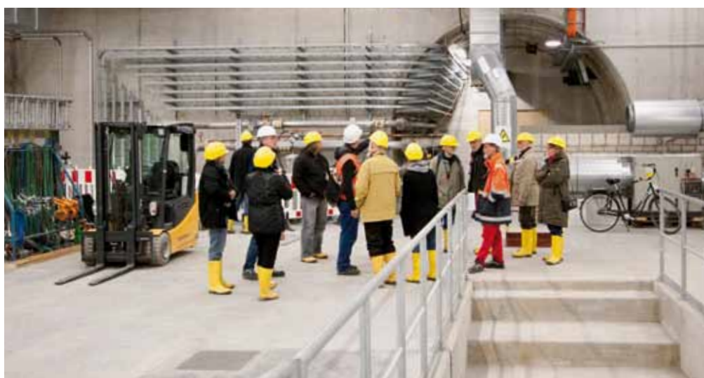
Figure 2 The group invited neighbours living near the Osdorfer Born construction site to special tours of the shaft building and tunnel.
