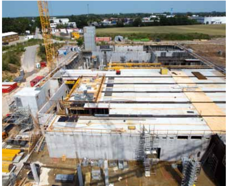
Figure 7 North view of the XHQ construction site (July 2014)
