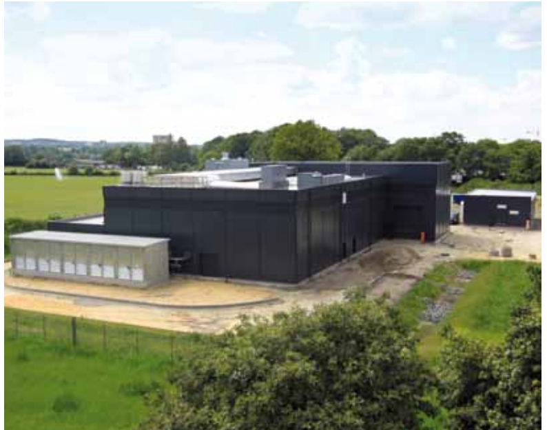
Figure 3 View from the eastern side of the building complex on the Osdorfer Born site (June 2014)
