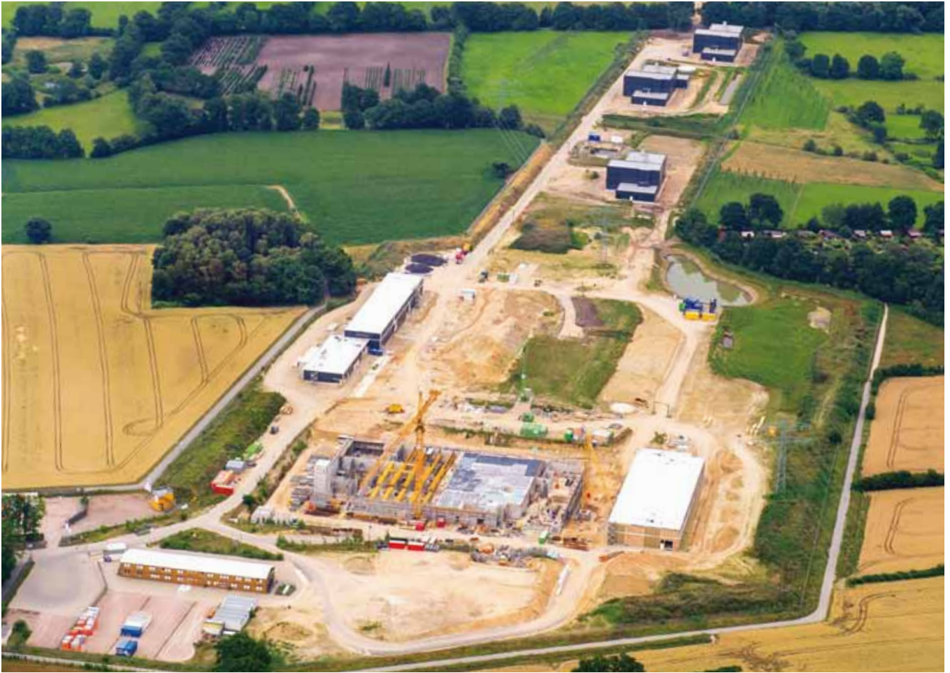
Figure 6 Aerial view of the entire Schenefeld construction site (July 2014)
