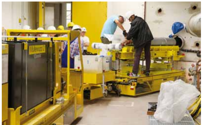
Figure 4 Installation of the injector dump (July 2014)
