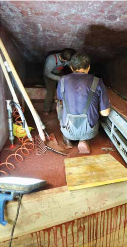
Figure 3 Pouring of heavy concrete into the injector dump pit (May 2014)
