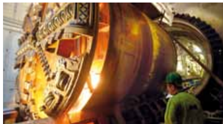
Figure 13 First tunnel boring machine after its arrival in the final shaft
