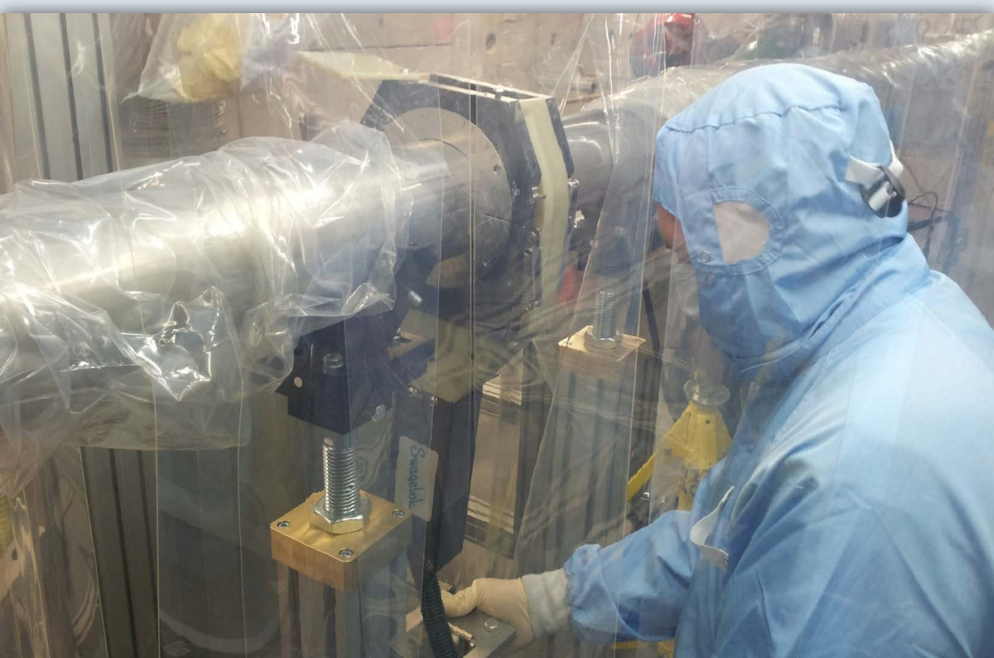
Figure 3. Orbital welding of UHV transport beampipes.
