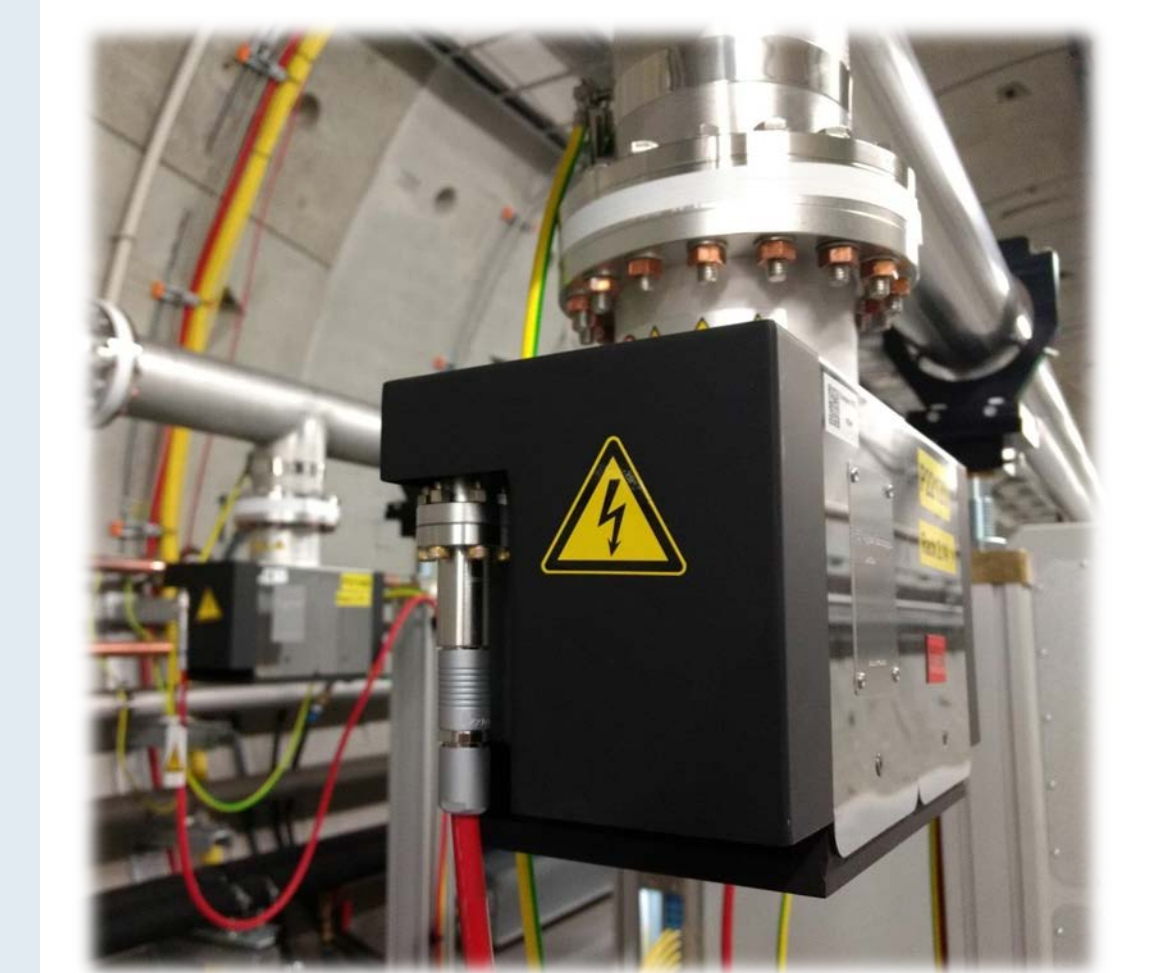
Figure 6. Examples of Triode Ion Getter Pumps installed in both branches of SASE2 Beamline.
